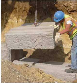
A block being set in place with a backhoe and chain.
